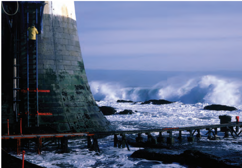
Above: Huge rollers break against the Inchcape Rock from the east. The iron walkways are seen to good effect in this shot. (Jim Bain)
